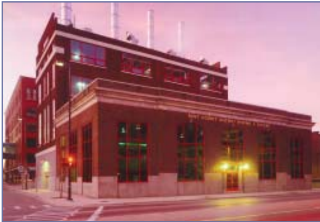
District Heating & Cooling Operations Building
