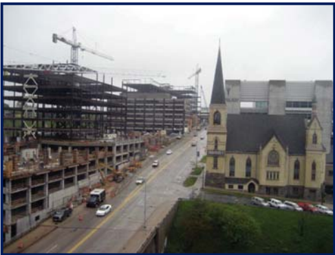
Michigan Hill Construction 2006 - 2007
