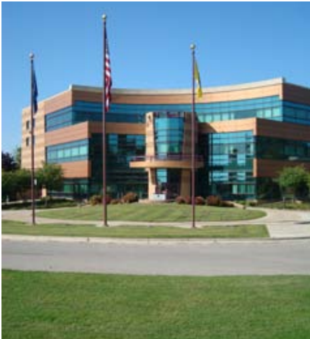
Sheriff Administration Building
