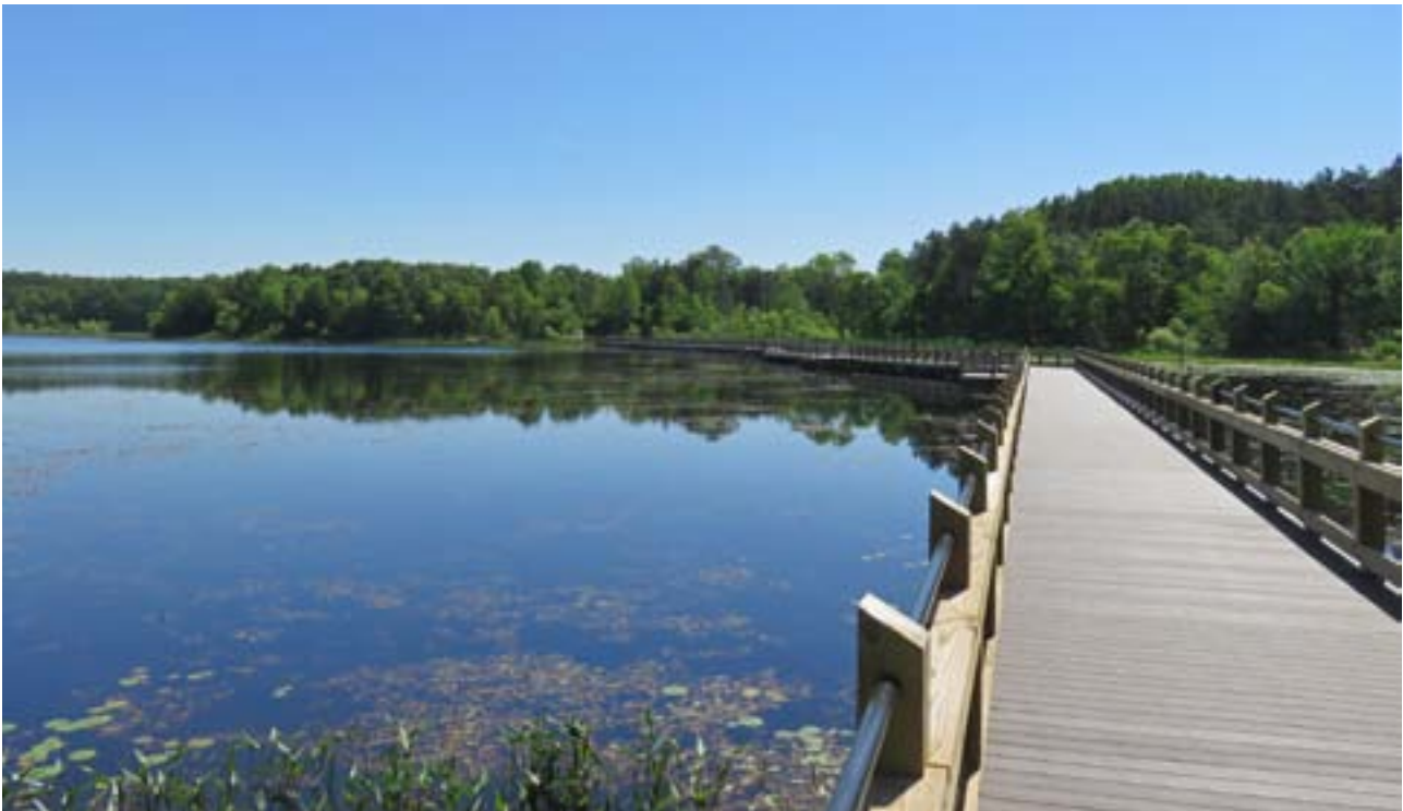
A project to install a new 900 ft boardwalk to replace the old floating boardwalk at Pickerel Lake Park was completed in 2016, with funding from the County's Capital Improvement Program and the Michigan Natural Resources Trust Fund.
