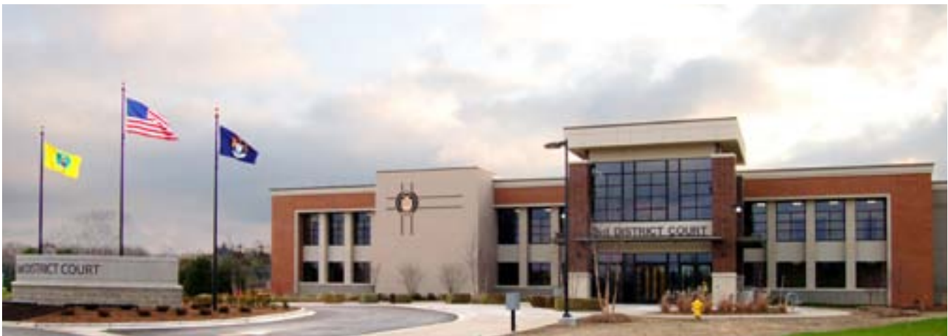
Kent County 63rd District Court facility
