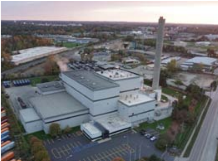
Kent County Waste to Energy Facility
