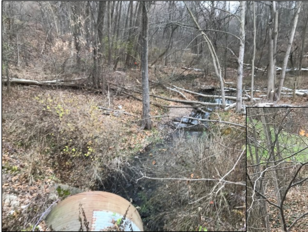
Woody debris, undersized culvert, erosion
