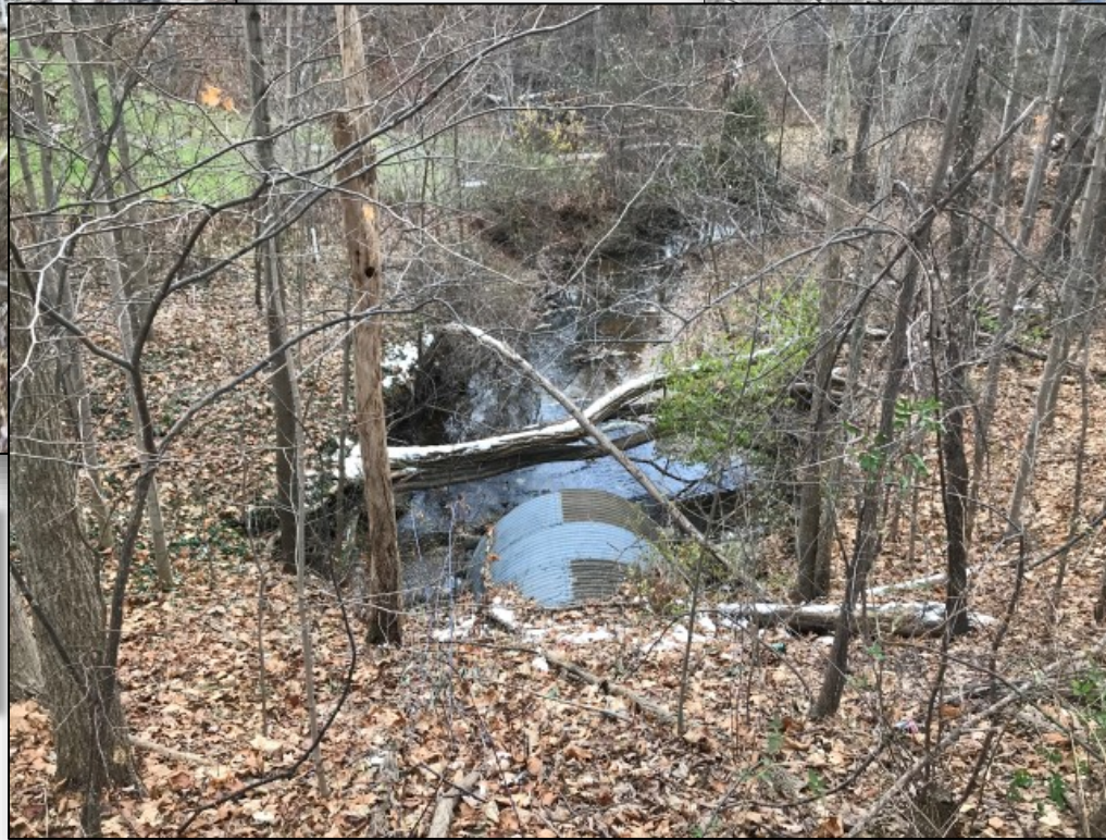
Woody debris, undersized culvert, erosion
